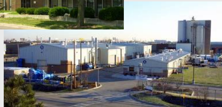
Energy & Environmental Technology Center
